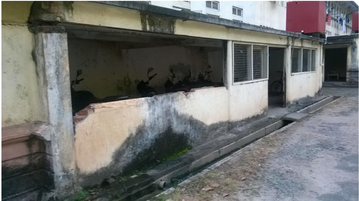
Existing cycle shed
