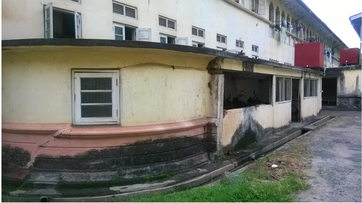
Existing cycle shed
